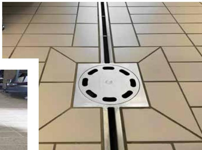
CANALE A FESSURA CON POZZETTO CON SCARICO VERTICALE
